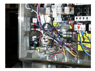
Showing the relay and time delay that control the start signal from the loader box start switch.
